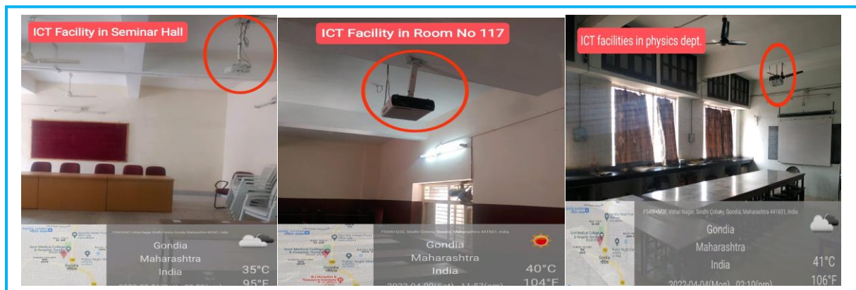
ICT facility in College
